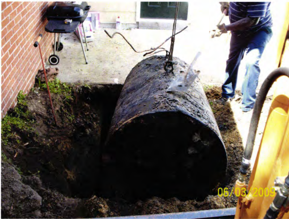
Picture 1: UST 1059Gardenia-1 during removal.
